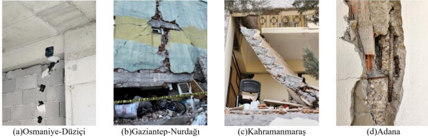
Fig. 27 Incorrect stirrup hook angle and buckling of longitudinal reinforcement
