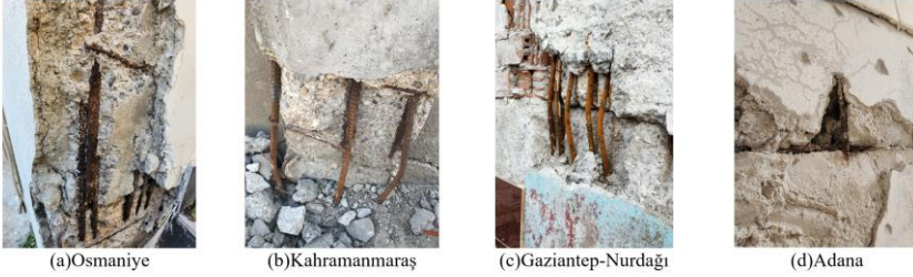
Fig. 25 Corrosion damages
