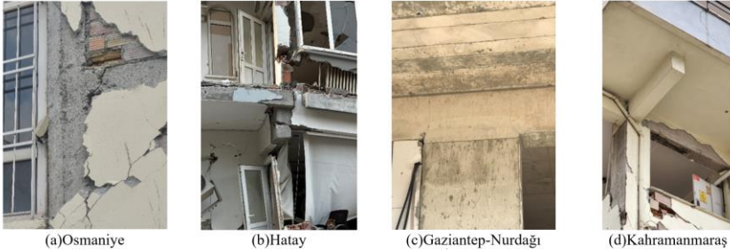
Fig. 23 Beam damages
