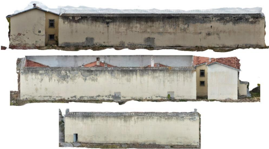
Figure 17 Orthographic Façades through Laser Scanning
