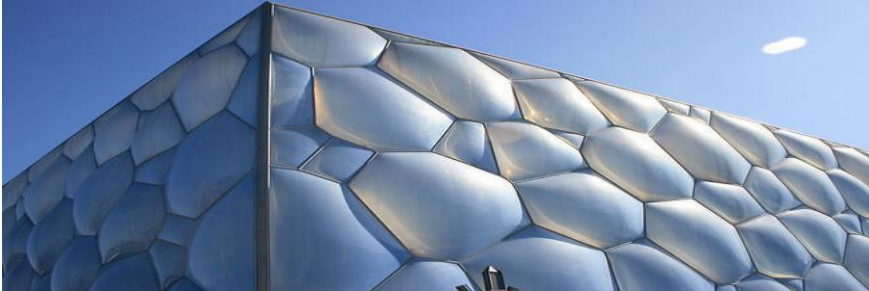
Image 1. ETFE Cushions Covering the Aquatic Centre
