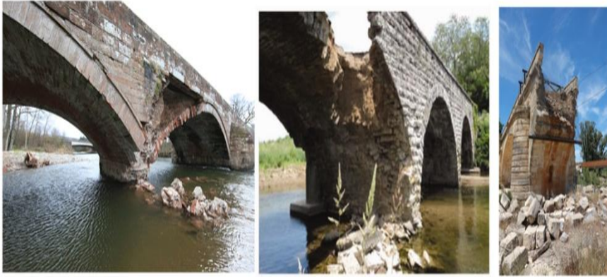
Figure 3 Examples of damaged stone bridges
