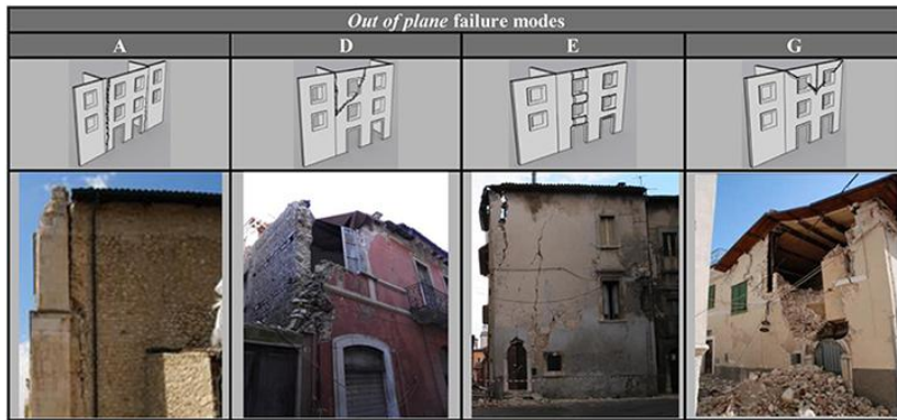
Figure 5: Out of plane failure modes
