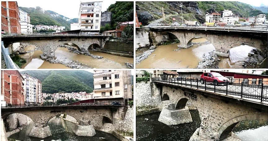
Figure 8 The historic Three-Span Bridge before it was demolished
