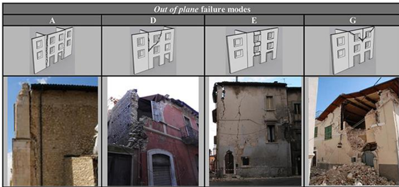
Figure 5: Out of plane failure modes
