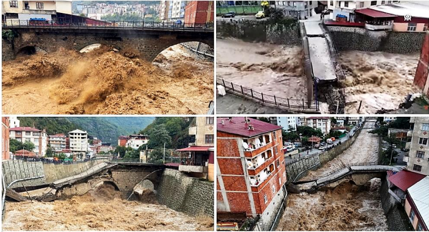
Figure 9 The historic Three-Span Stone Bridge after its collapse
