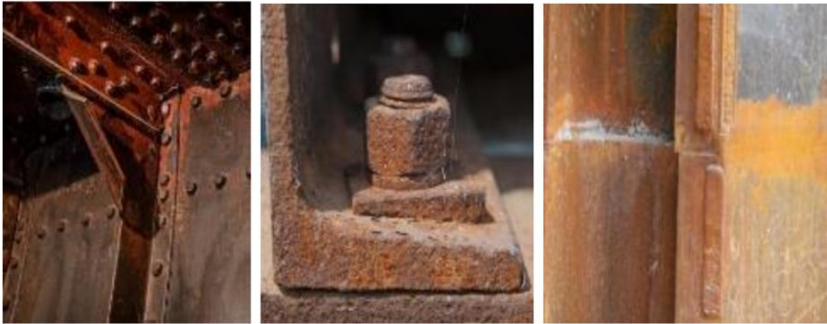
Figure 2: Methods of Joining Steel Components
