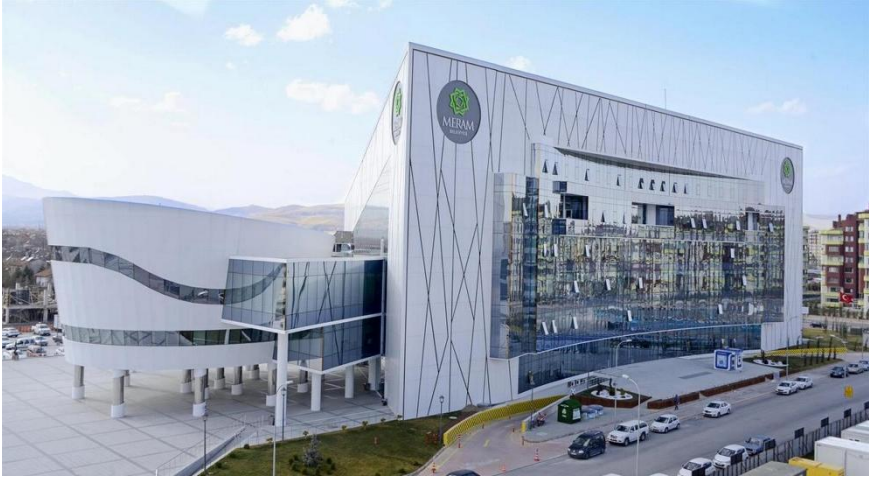
Figure 10 Konya Meram Municipality Building (KMMB)
