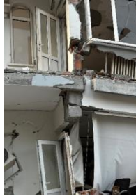
Figure 23 Beam damages
