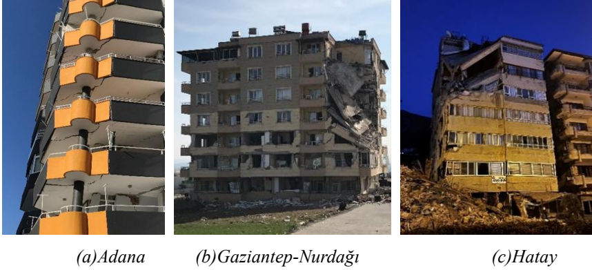
Figure 19 Corner column damages
