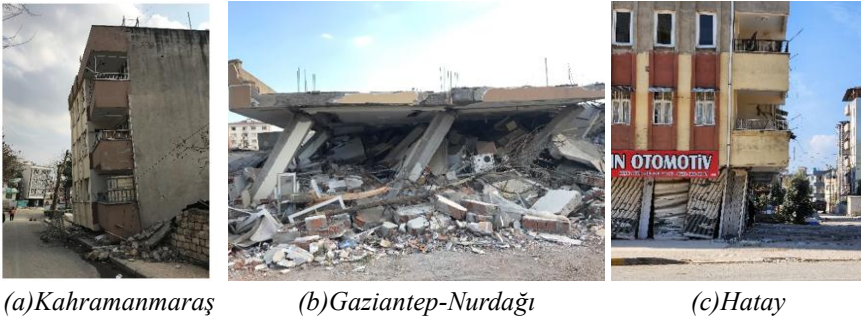
Figure 11 Observations of damage due to soft/weak story irregularity
