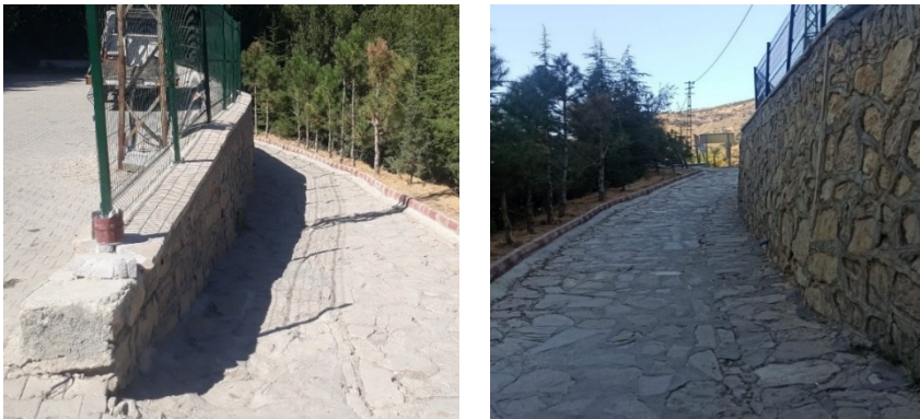
Figure 7. Retaining Wall at the Entrance to the Area
